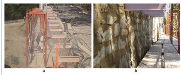
Figure 8: Holes and cracks cleaning and filling (Conde Salazar, 2007).
