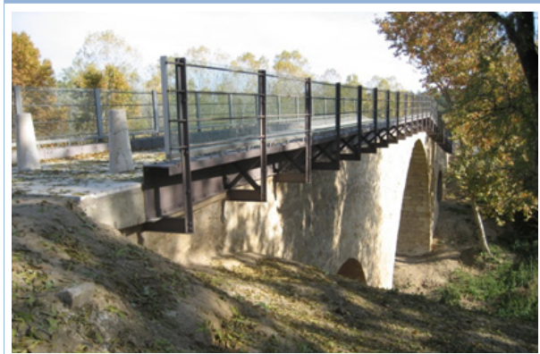
Figure 9. Bridge status after restoration. (Conde Salazar, 2008)
